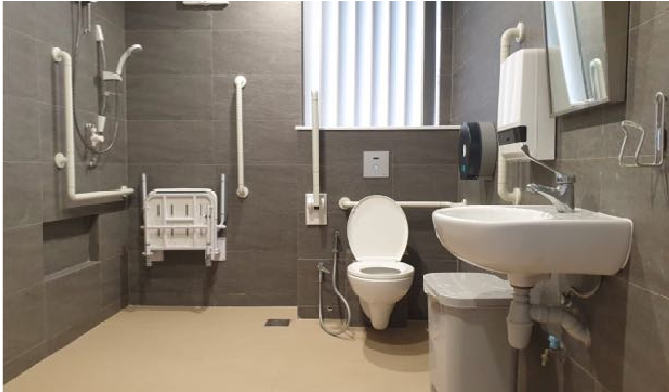
Application of colour contrast – white fixtures against coloured background tiles.
