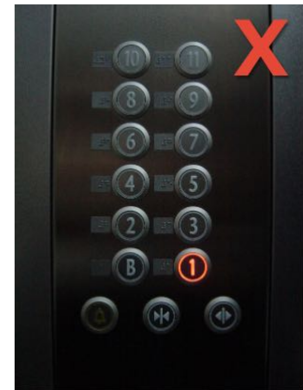
Buttons with insufficient contrast
